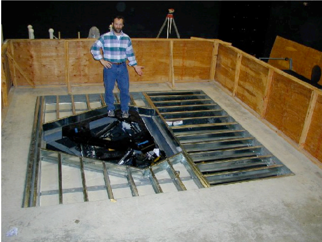
ACITC 3 rd floor: framing prior to cement board
