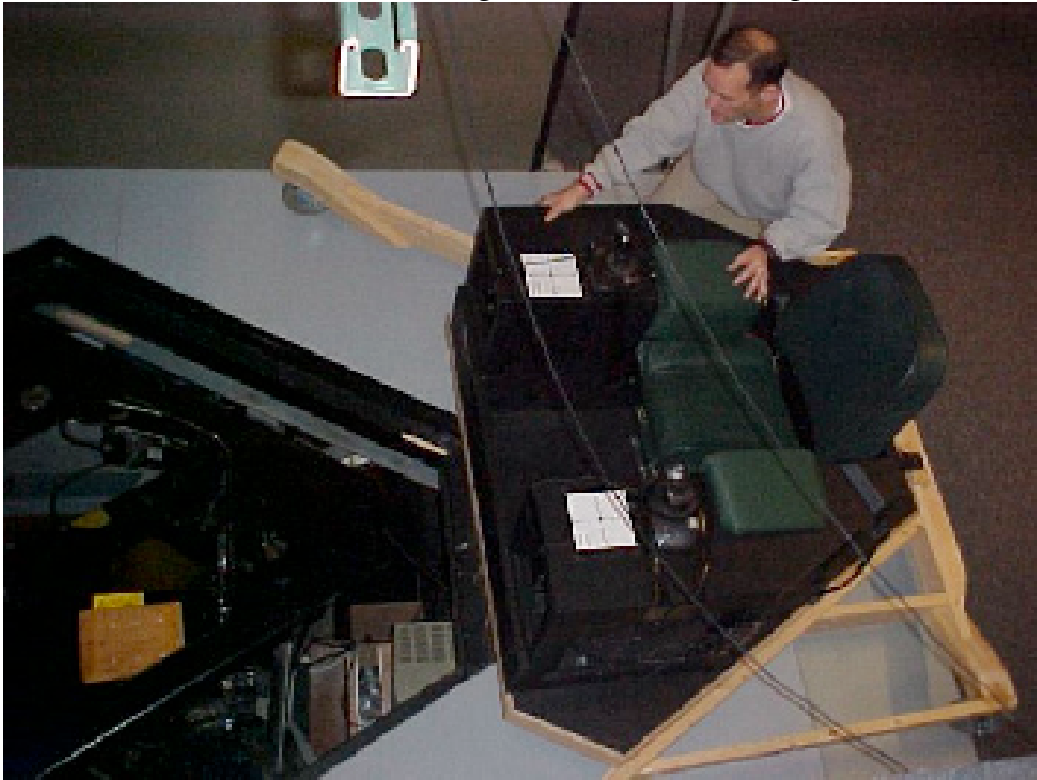
ACITC 3 rd floor: installing chair: bolt chair onto motion platform
