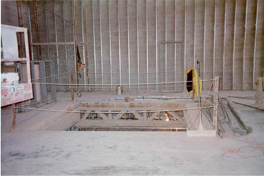
ACITC 3 rd floor: CAVE floor substructure under construction
