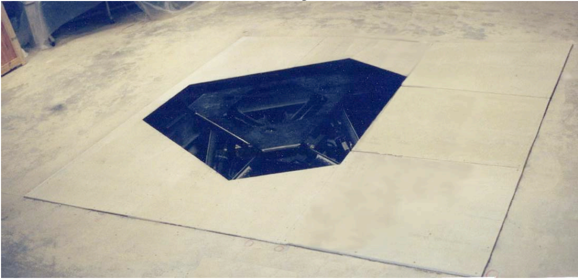
ACITC 3 rd floor: framing with cement board
