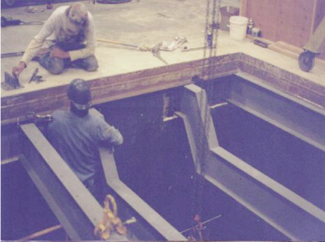
ACITC 3 rd floor: CAVE floor substructure under construction
