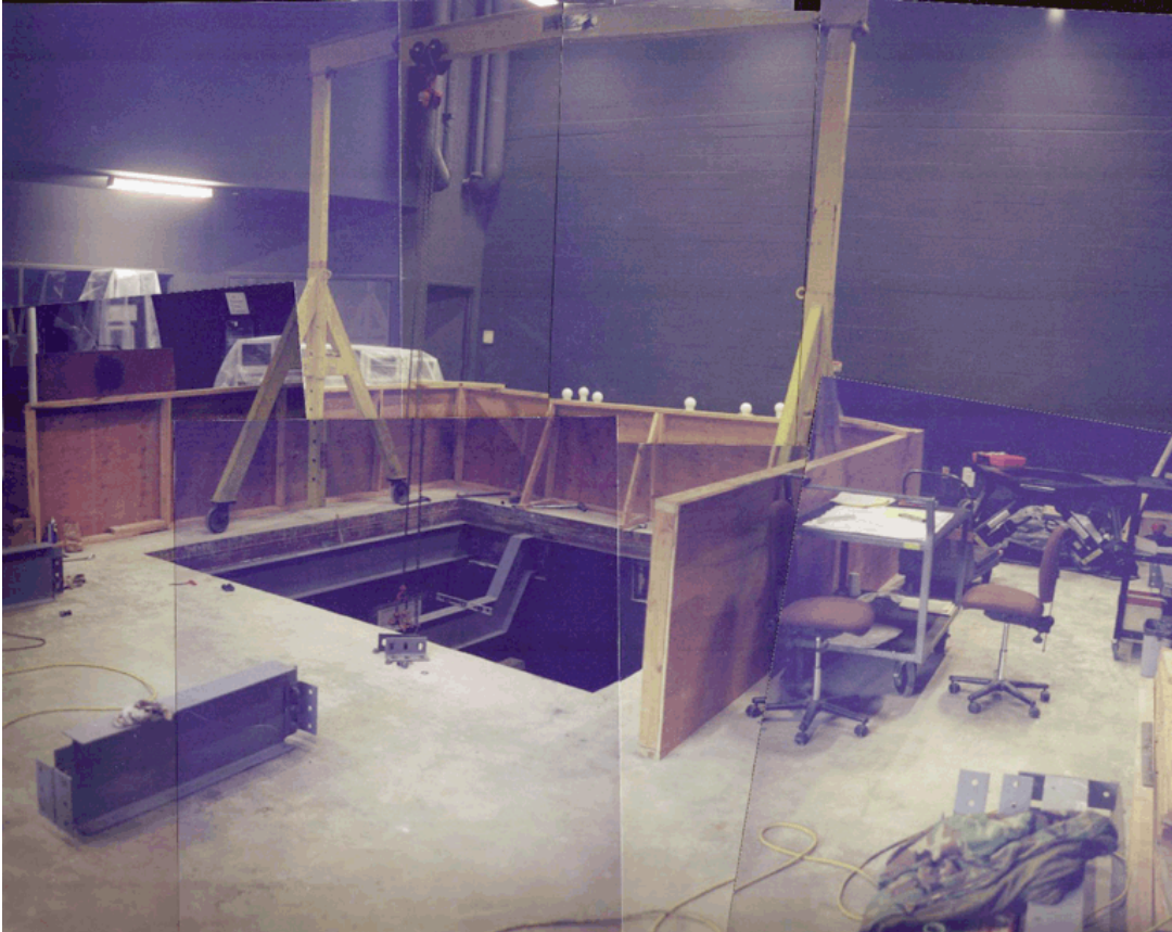
ACITC 3 rd floor: CAVE floor substructure under construction
