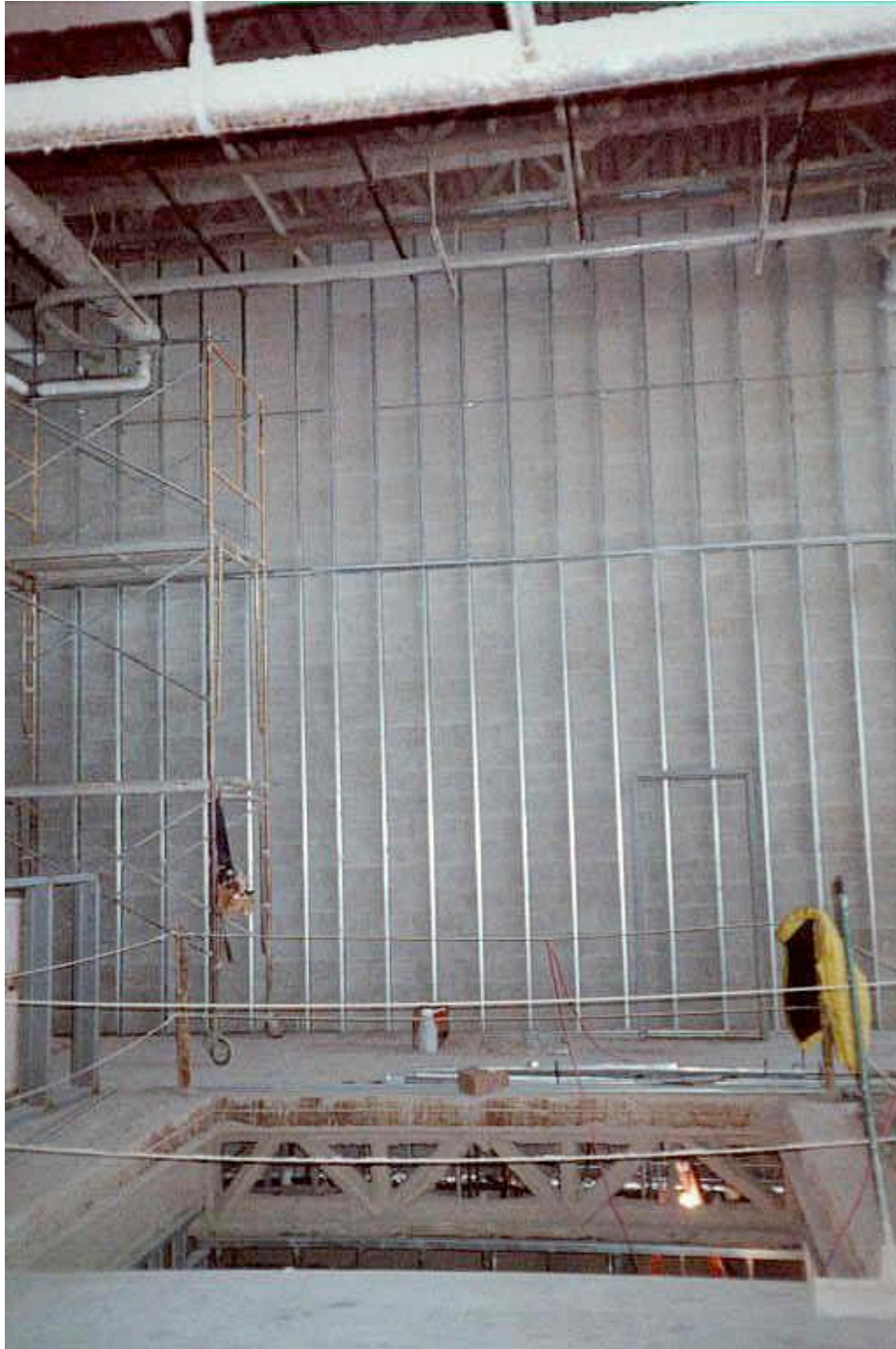
ACITC 3 rd floor: CAVE floor opening under construction, tall view
