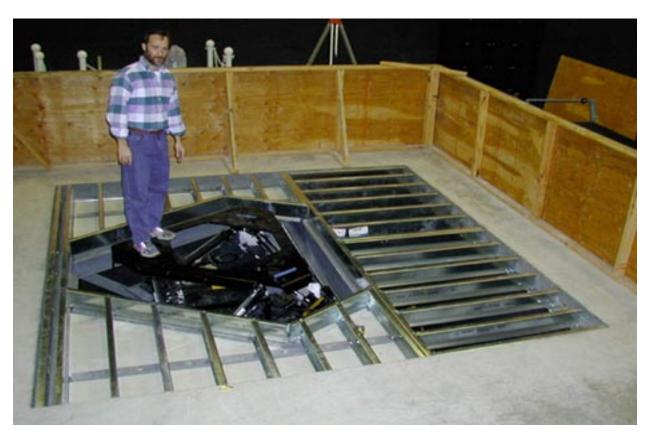
Figure 4. CAVE floor substructure and motion base under construction, February 13, 2001.
